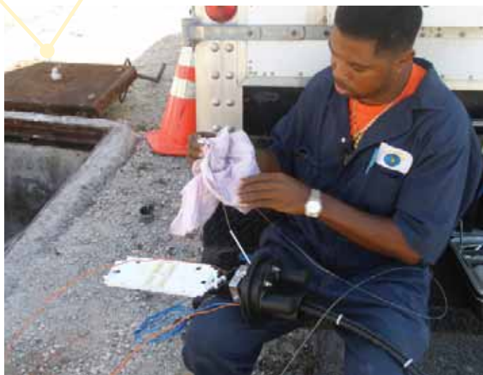
BTC technicians at work
